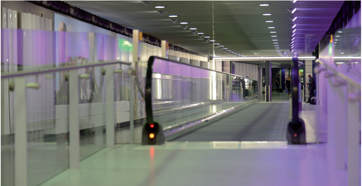
Pasillo rodante (iwalk) en Heathrow Airport, Londres.
